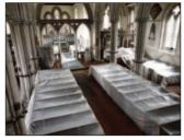
The first move was to envelop pretty well everything above ground in Holy Trinity in plastic sheeting - an A-grade packaging job. This was followed by moving the pews in the N aisle to the rear of the nave, removal of the rotten and dry rot infected flooring, joists and the boarding (dado) along the North wall. The solid supports for the joists were also removed. (I don't know how he did it,
